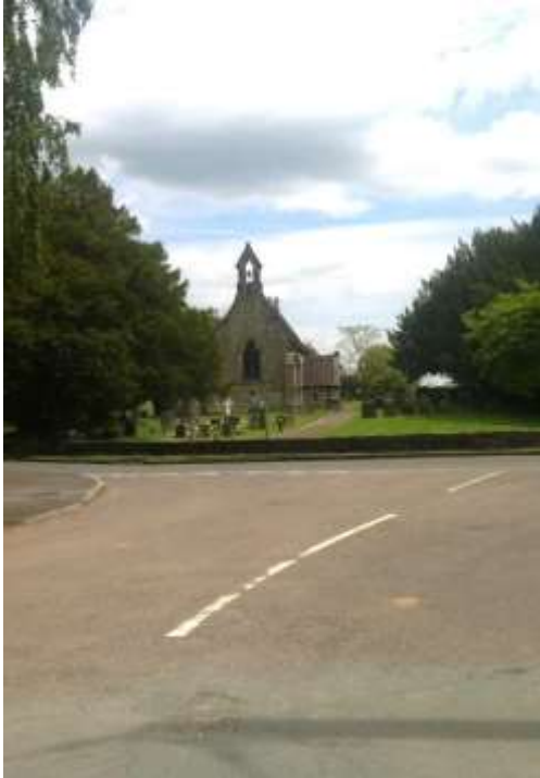
Figure 58 Specific view of St. John the Baptist Church
