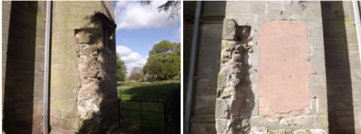
Figure 62 Poor condition of stonework and poorly executed patch repairs to The Gatehouse masonry
