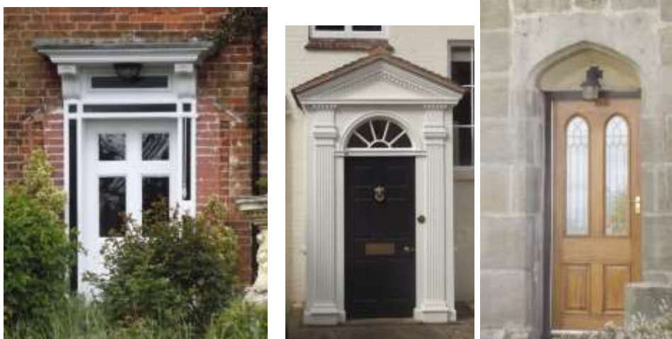
Figure 22 Doorways of the conservation area reflect Georgian and late Medieval period style
