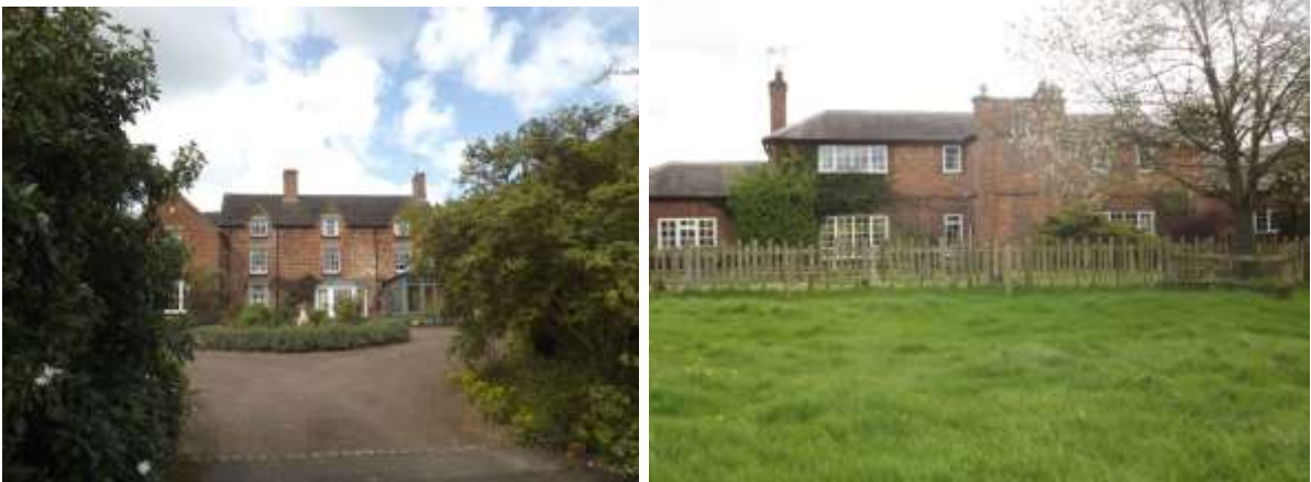
Figure 40 Tixall Farmhouse and Kennels Farm
