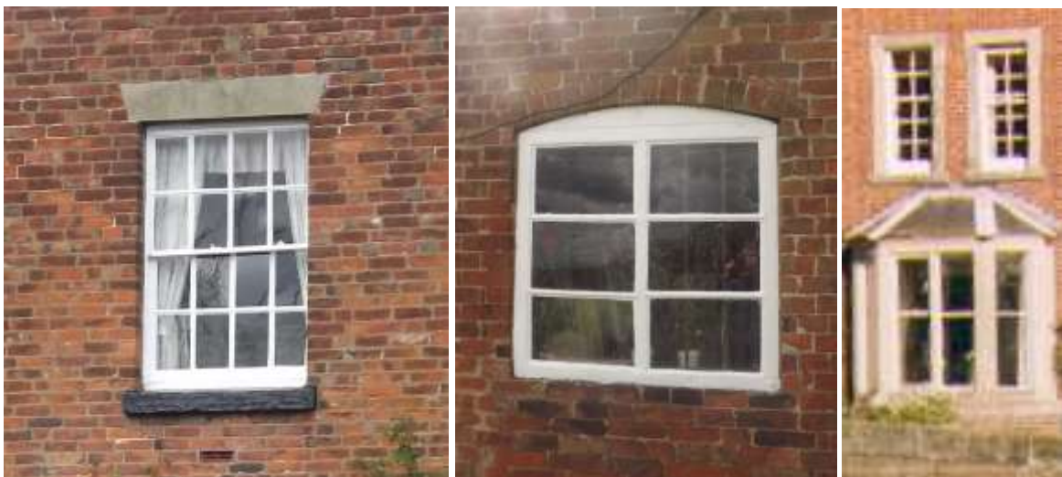
Figure 20 Sliding sash windows and pegged fixed casement at Tixall Farm, and stone surrounds and frames at Tixall Lodge
