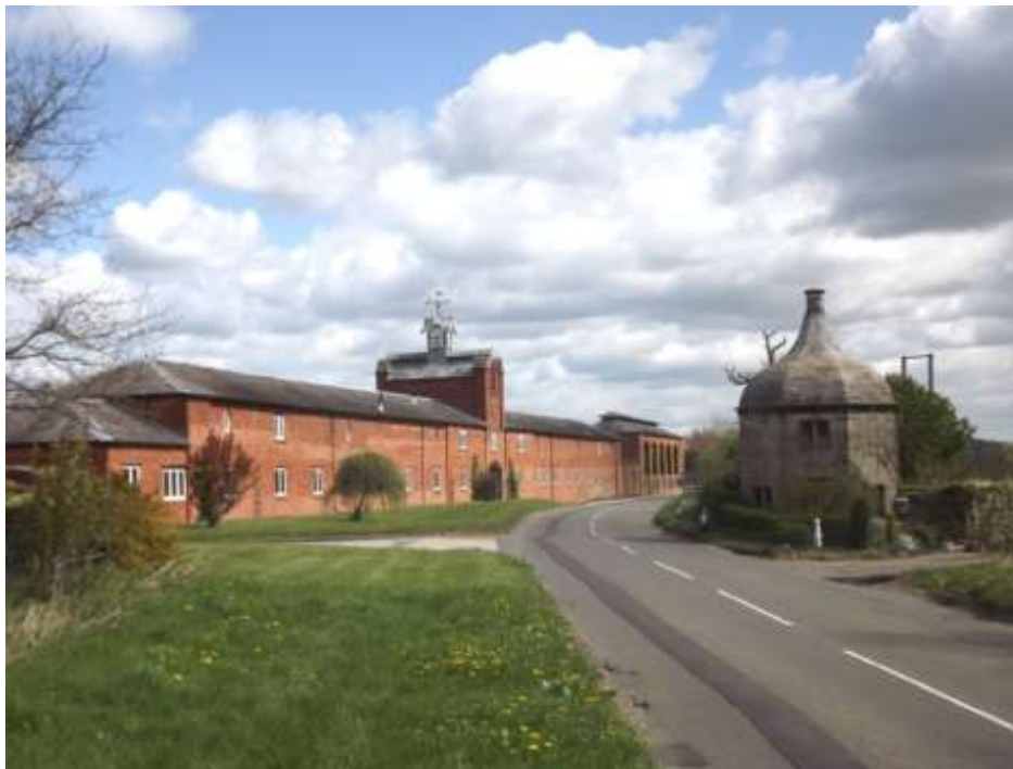
Figure 31 Bottle Lodge and Tixall Farm Buildings create a contrast in the landscape in terms of scale and building materials
