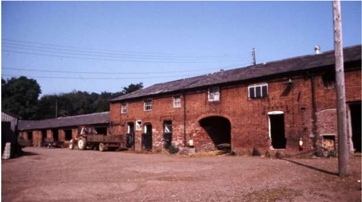
Figure 13 Tixall farm buildings in the 1980s prior to residential conversion (Reproduced with permission from Anne Andrews)
