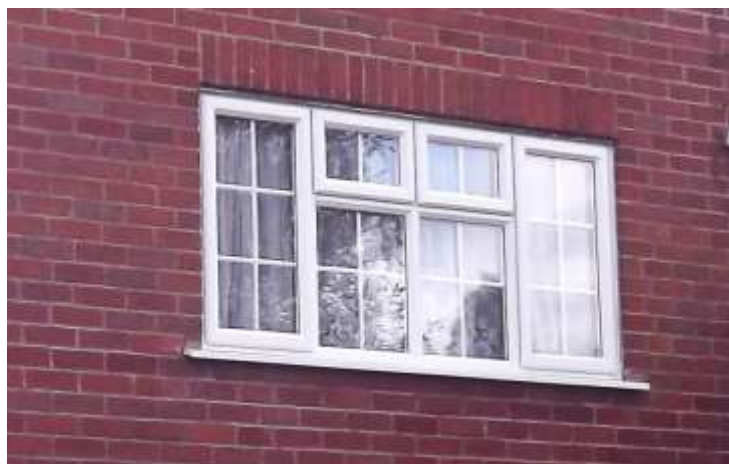
Figure 61 uPVC windows and the use of modern red brick laid in stretcher bond
