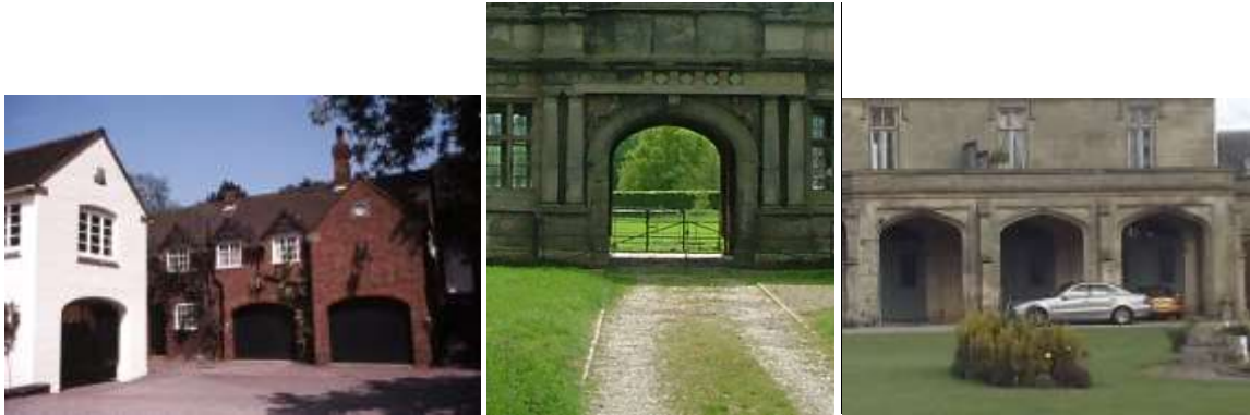
Figure 23 Coach and cart style openings feature throughout Tixall
