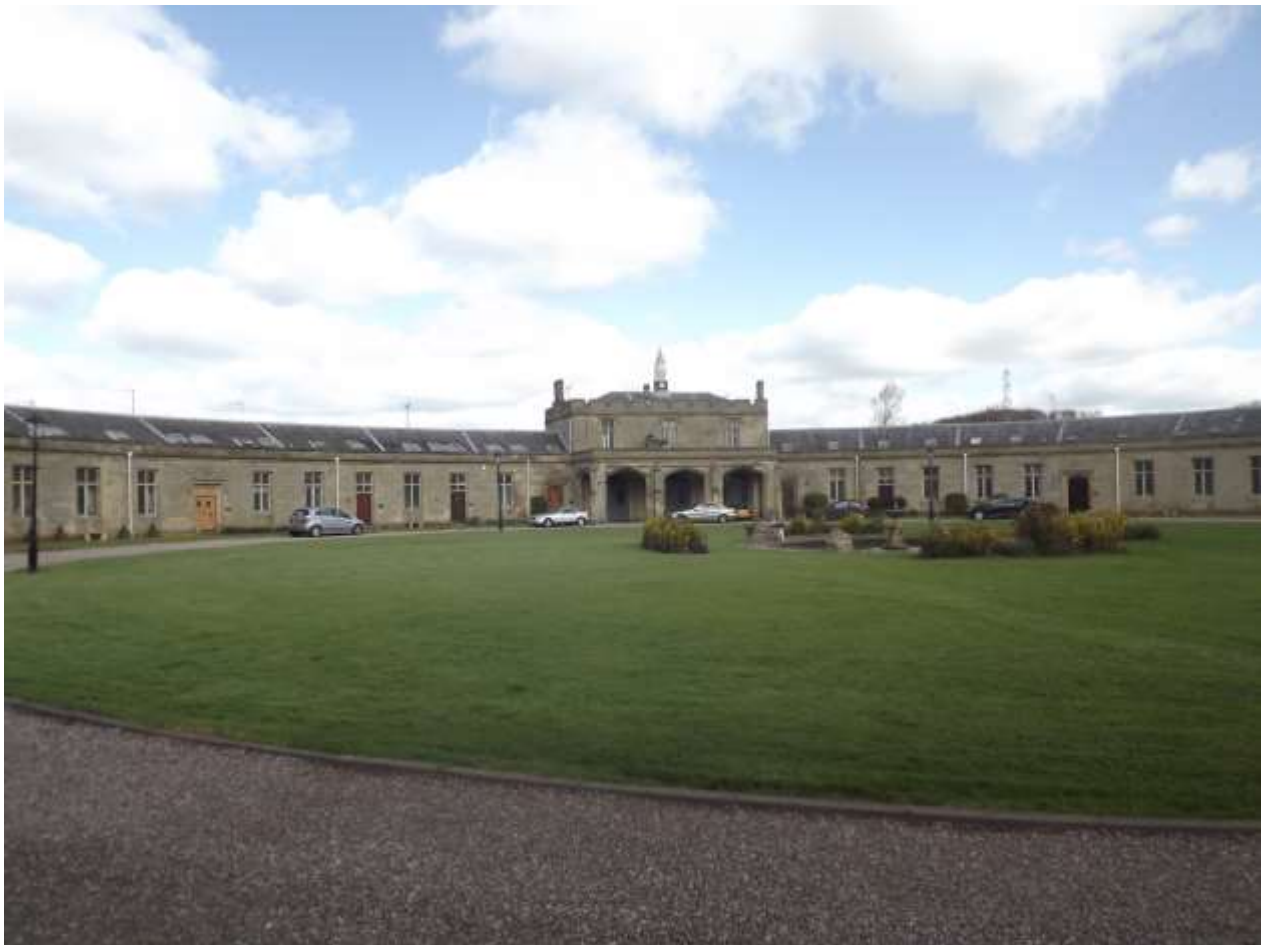
Figure 28 Tixall Mews is a semi-circular former stabling and coach house
