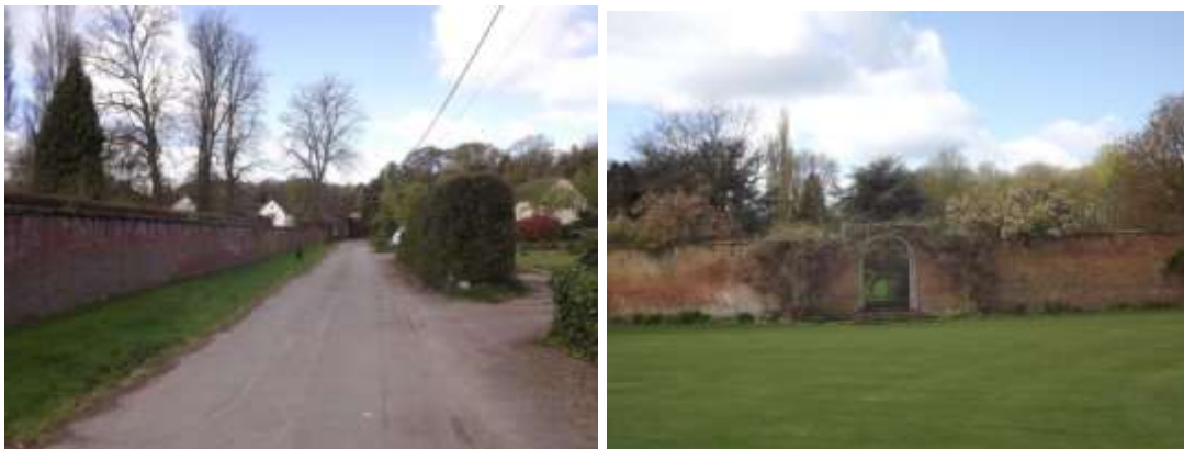
Figure 50 High brick walls form important boundaries in Tixall
